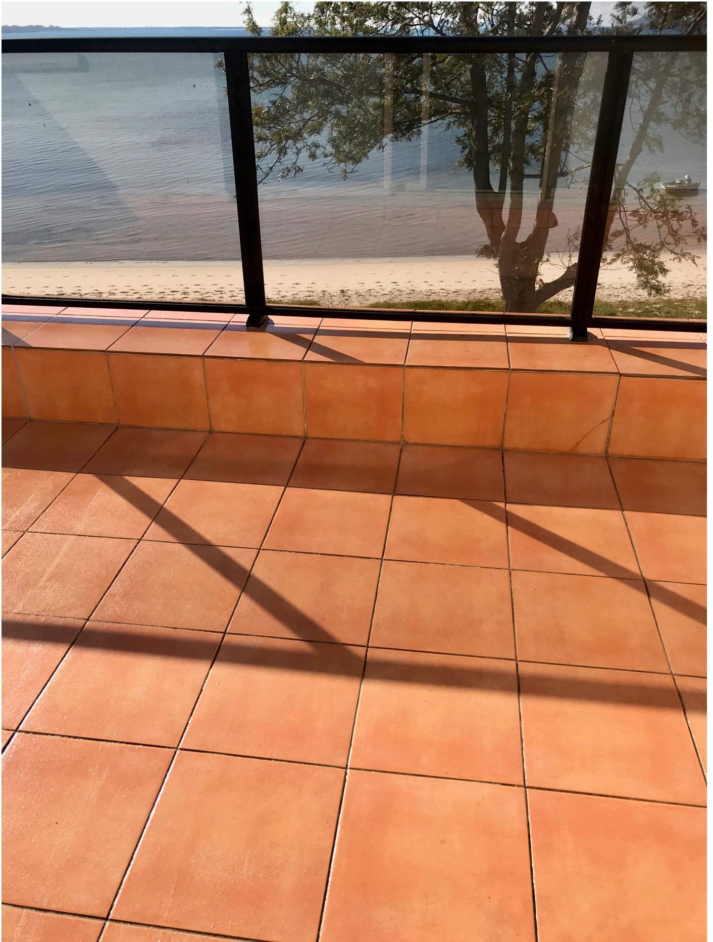
Clear Waterproofing Membrane installed over tiles
